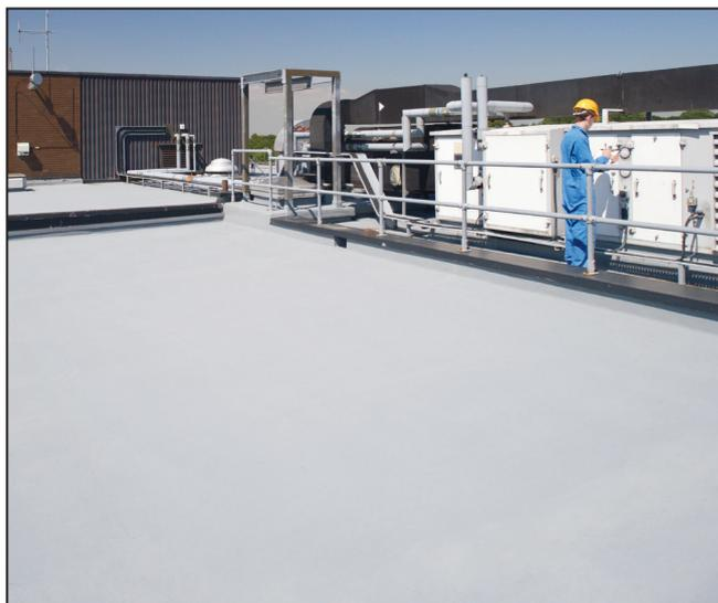
Above: Elastaseal™ Z used on the roof of a food processing factory.
