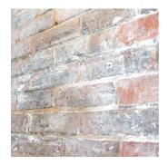
Watco Masonry Waterproofer looks white immediately after application, so it is easy to tell which areas have not been treated.
