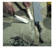
Joint sides should be clean and dry. Spalled joints should be repaired initially using Watco Concrex. (For best results use Watco Back Up Rod to reduce deeper joints to the desired depth.)
