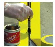
Apply primer by brush to the sides of the joint and allow to dry (approximately 30 minutes at 20°C). Masking tape may be used.
