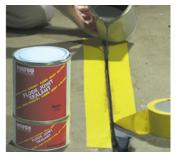
Crimp the rim of the tin to facilitate pouring and pour evenly into the prepared joint, leaving the top of the joint sealant just below the surface of the floor.
