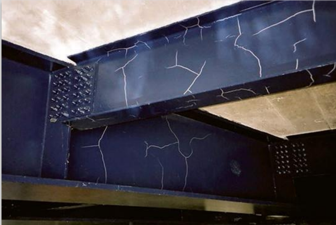
Fig. 16 Similar to checking but the cracks are generally wider and penetrate deeper into the film.
