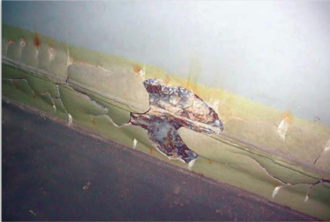
Fig. 14 The splitting of a dry paint film through at least one coat to form visible cracks, which may penetrate down to the substrate. Cracking comes in several forms, from minute cracking to severe cracking.
