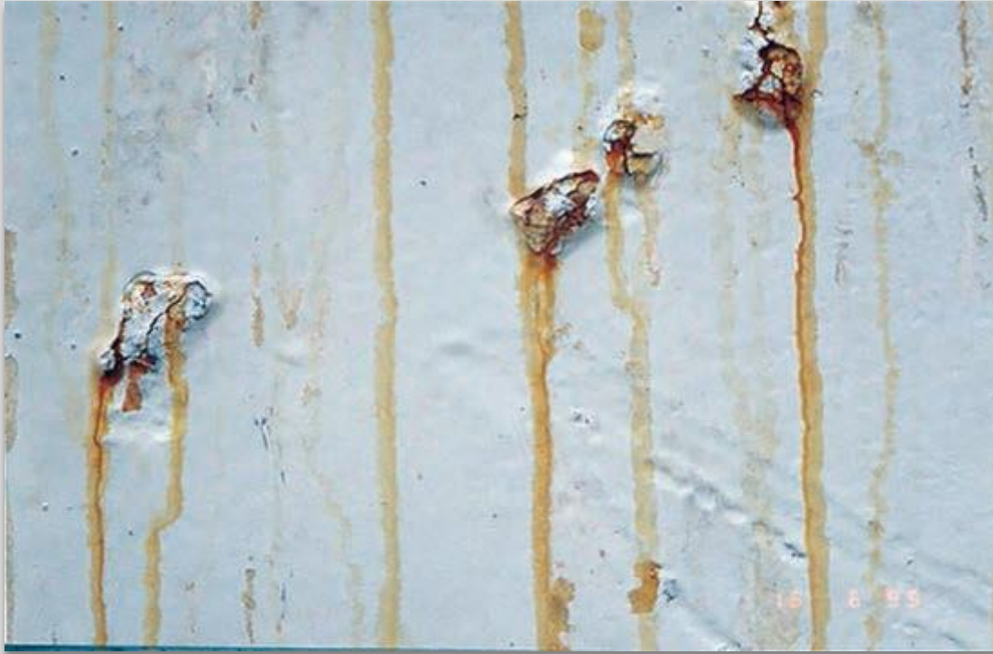
Fig. 33 A light staining on the surface of the paint caused by the precipitation of ferrous oxide from adjacent exposed steel.
