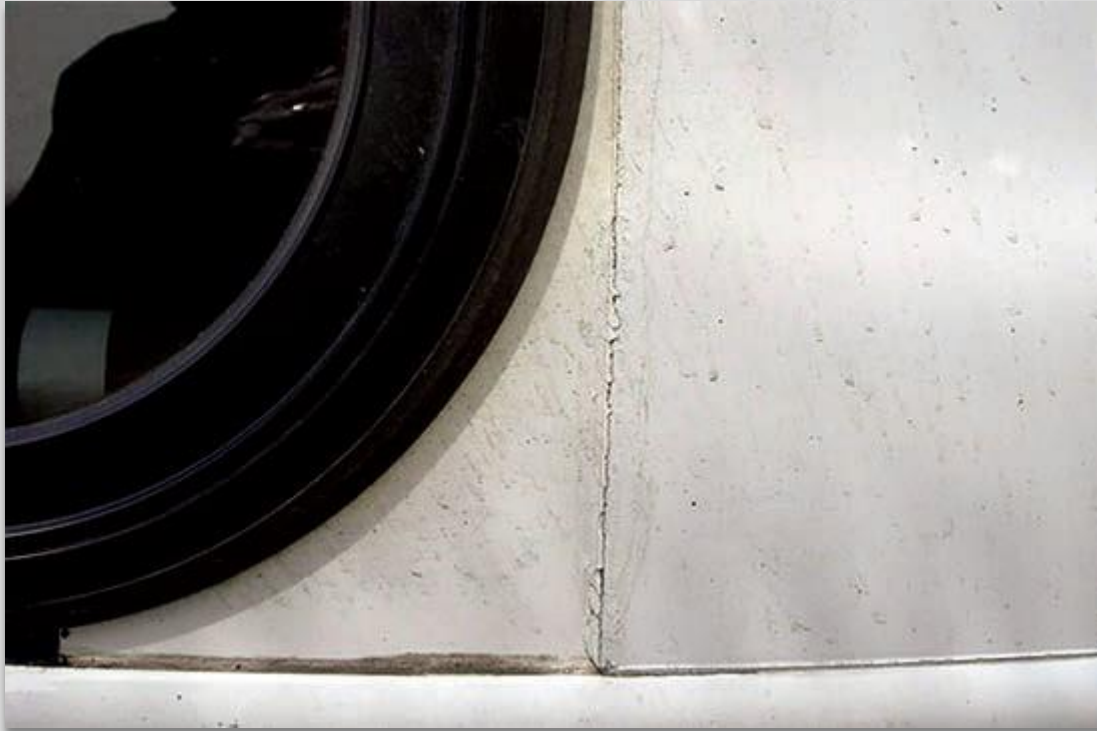
Fig. 7 The covering over of unfilled gaps such as cracks or corners with a film of coating material. This introduces a weakness in the paint film, which may crack or flake off.
