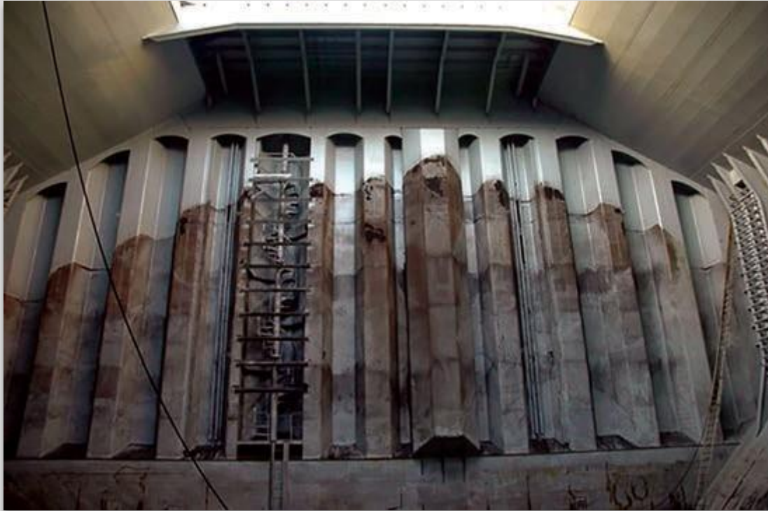
Fig. 39 Discoloration of a coating system.
