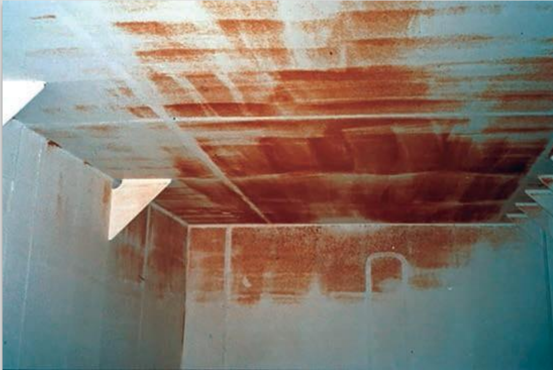
Fig. 31 Fine spots of rust that appear on a paint film, often a thin primer coat. The initial spots rapidly spread over the surface, resulting in a film of rust through which the individual spots are difficult to discern. Also from holidays.
