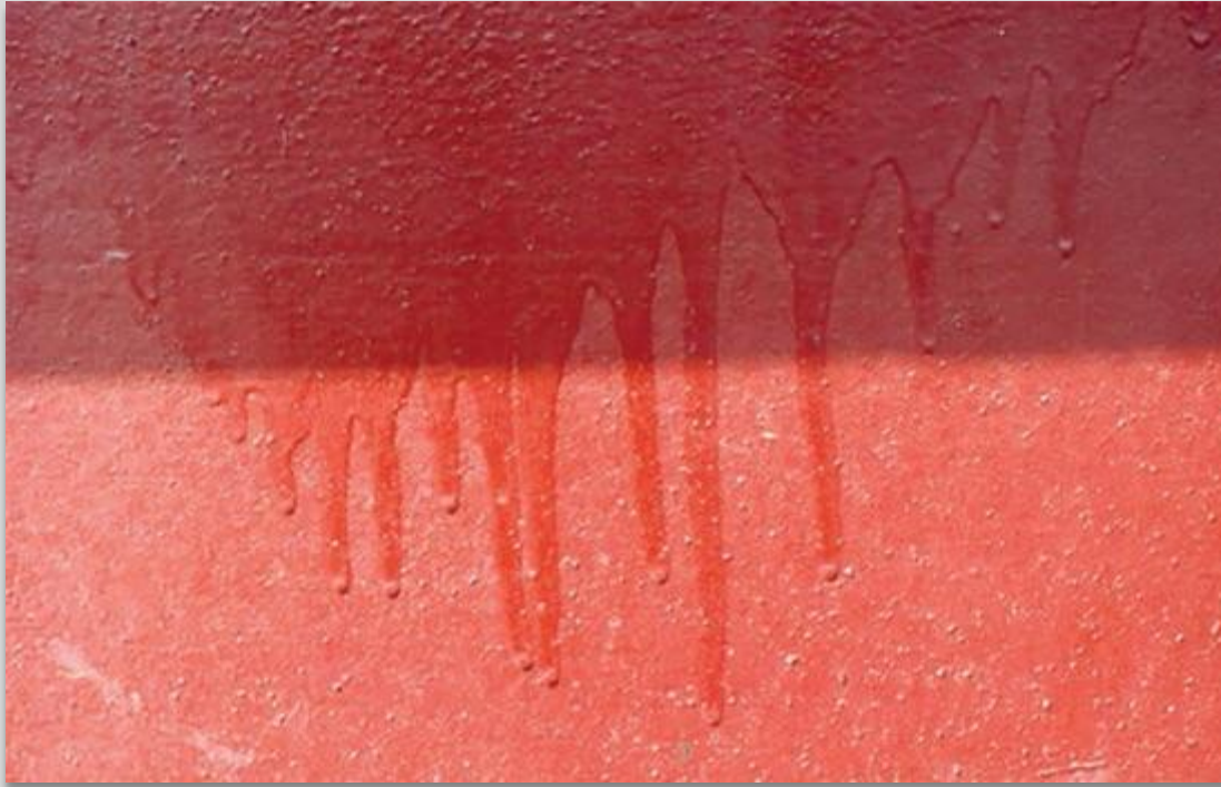
Fig. 30 A narrow downward movement of a coat of paint, often apparent from accumulation of excessive quantities of paint at irregularities such as cracks and holes where the paint continues to flow after the surrounding surface has set.
